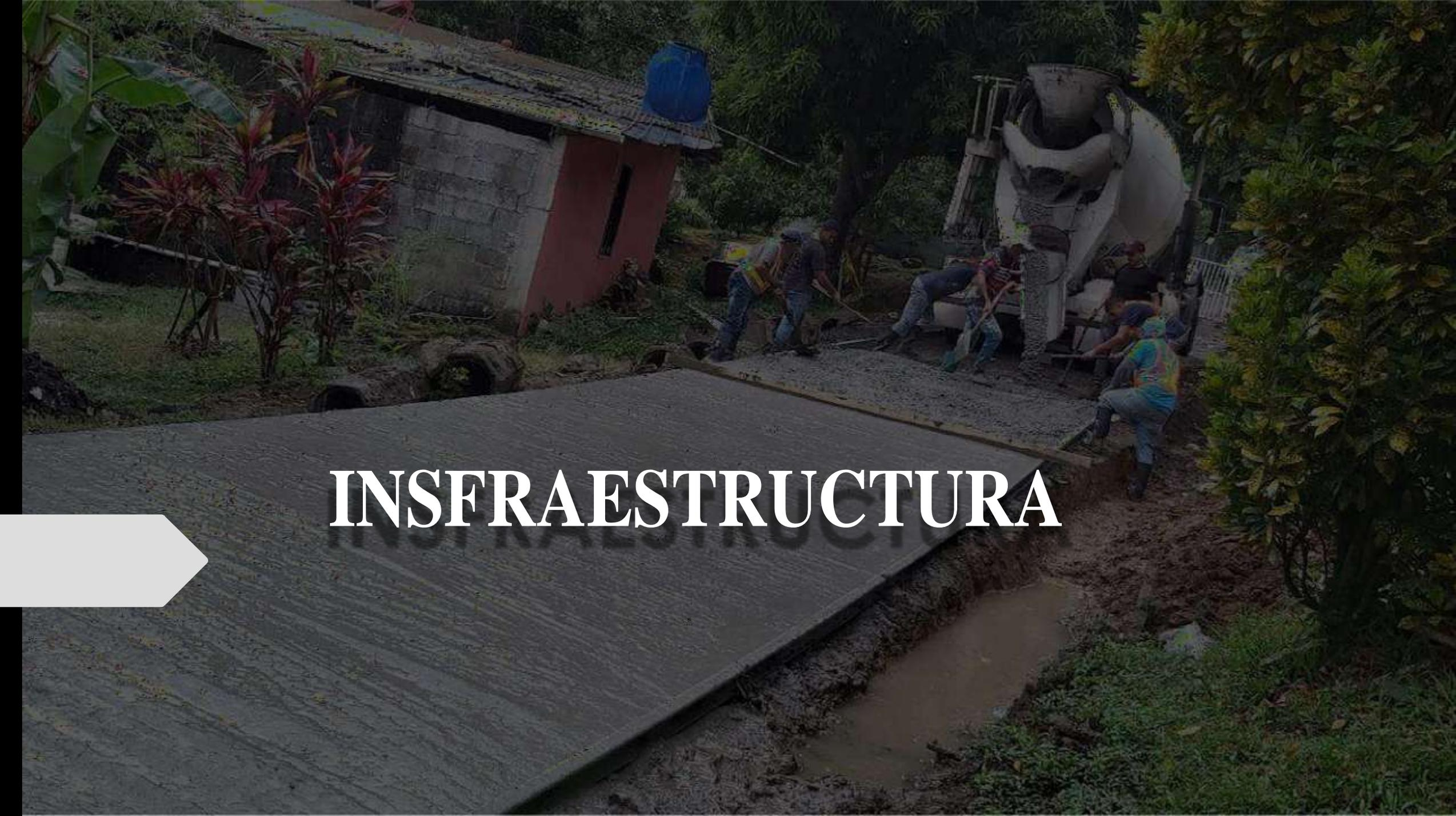
A photograph of a construction site in a rural area. A concrete mixer truck is parked on a dirt path, pouring concrete into a prepared trench. Several workers in colorful shirts are using tools to guide the concrete. In the background, there is a small building with a corrugated metal roof and a blue water tank. The scene is surrounded by lush greenery and trees.
